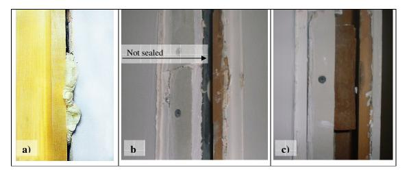
Figure 3– Example of the use of flexible foam and small pieces of wood to fix doors. Font: a) Manufactures catalogue b,c) photos by the author.
