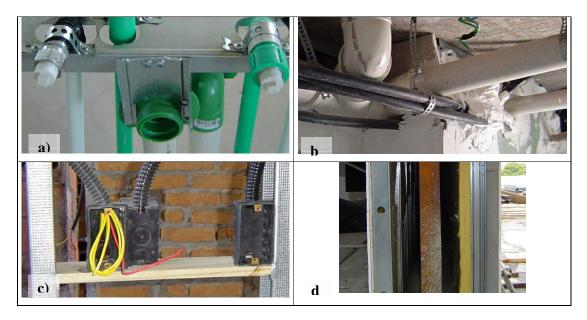
Figure 4 – Examples of sound transmission paths found: a) pipes with no resilient isolation; b) pipes glued to gypsum board walls; c) back-to-back electrical outlets in the same structure; d) better sound insulation performance of gypsum wall.
